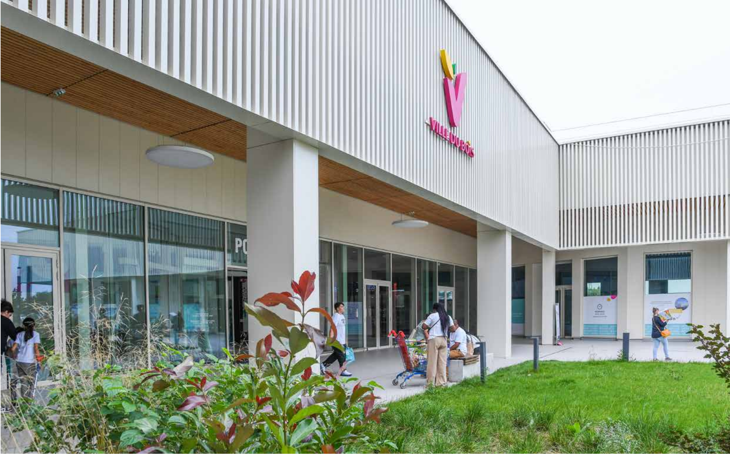
Centre commercial La Ville-du-Bois (91)
